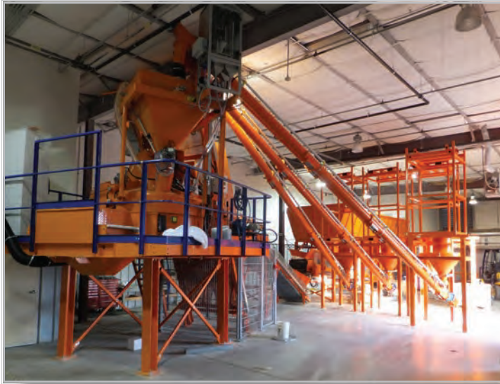
CTIS Concrete Batching Plant
