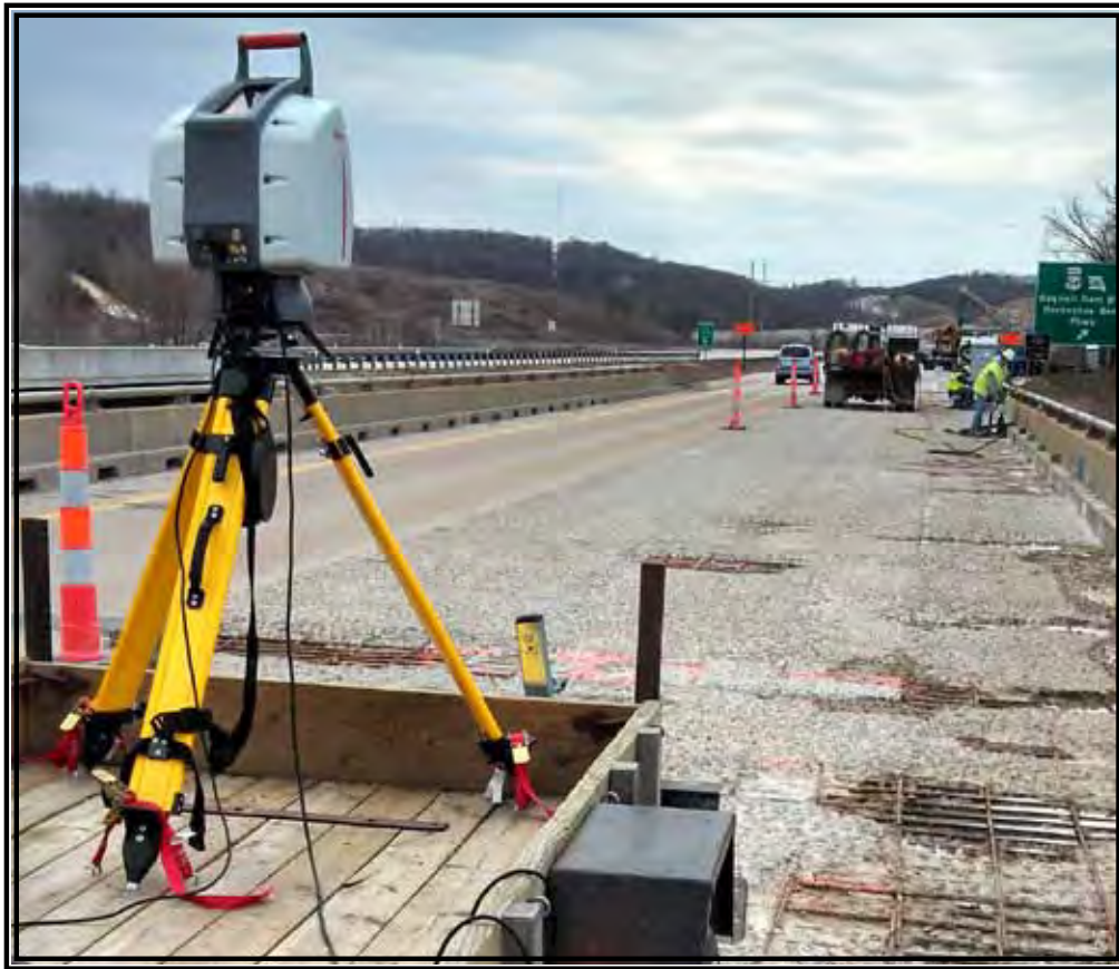
Figure 1. LIDAR scanner set up to scan a Missouri bridge after hydro-demolition used to remove unsound concrete
