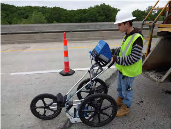
Figure 1. Ground Penetrating Radar Unit Scanning Bridge Deck
