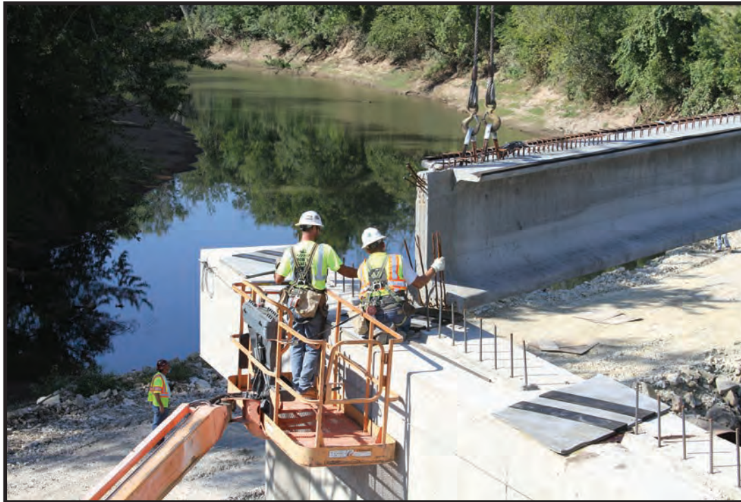
Figure 2. Bridge girder with instrumentation being set.
