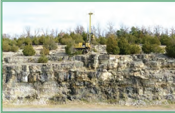
Figure 1. Drilling and installing monitoring wells on the south site.
