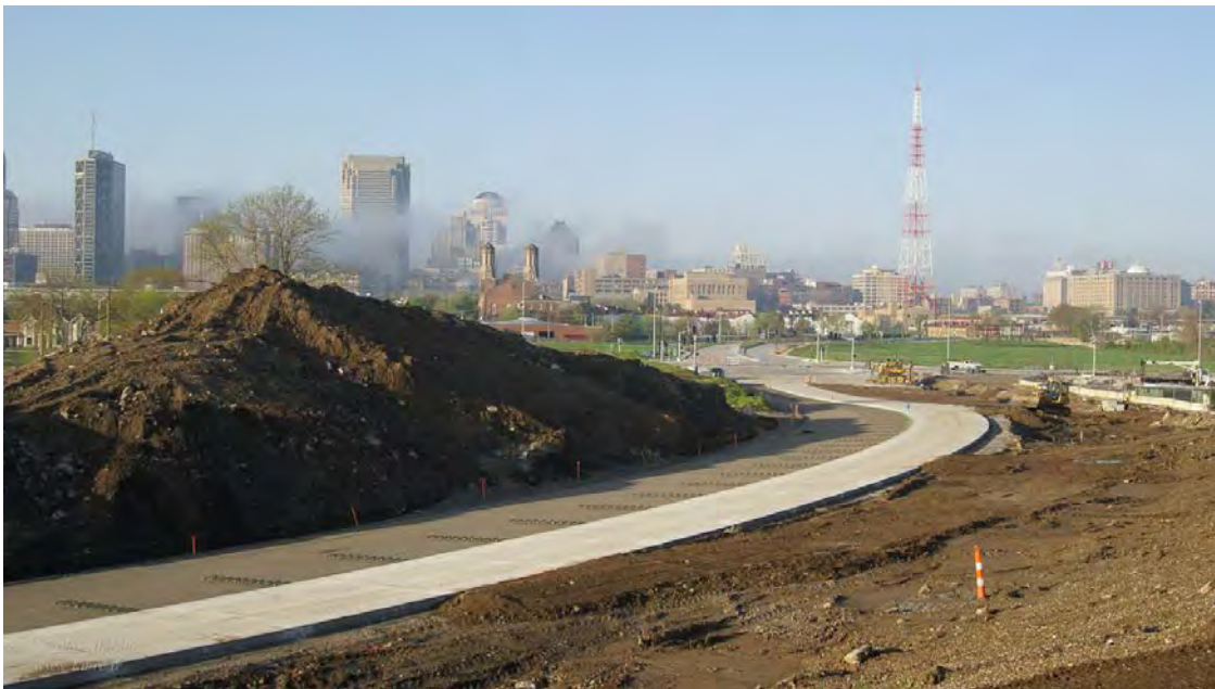
Figure 1. General View of the Ramp Approach with the Reference Section Already in Place
