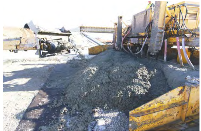
Figure 2. Casting pavement sections with RCA-made concrete
