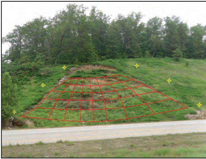
Figure 2. Test site in landslide in Branson MO. Rebar with 4” targets will be positioned on yellow markers (outside of the slide) for control, and at each intersection of the grid within the slide.
