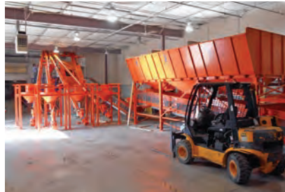
New concrete batching plant
